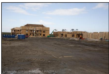
Framing for the residential complex
